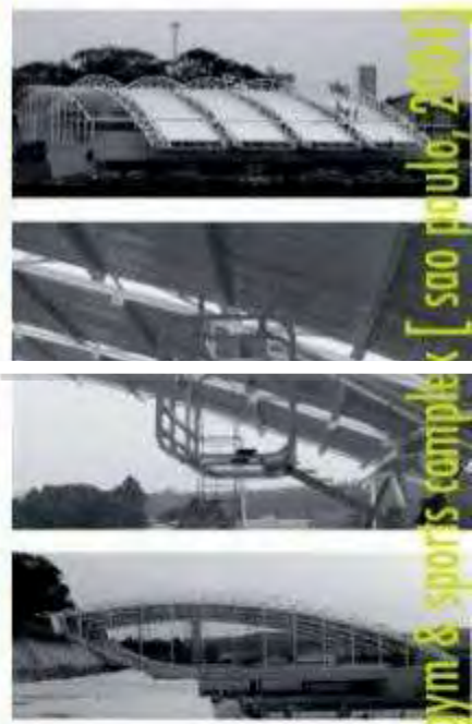
[construction in September 2004]
